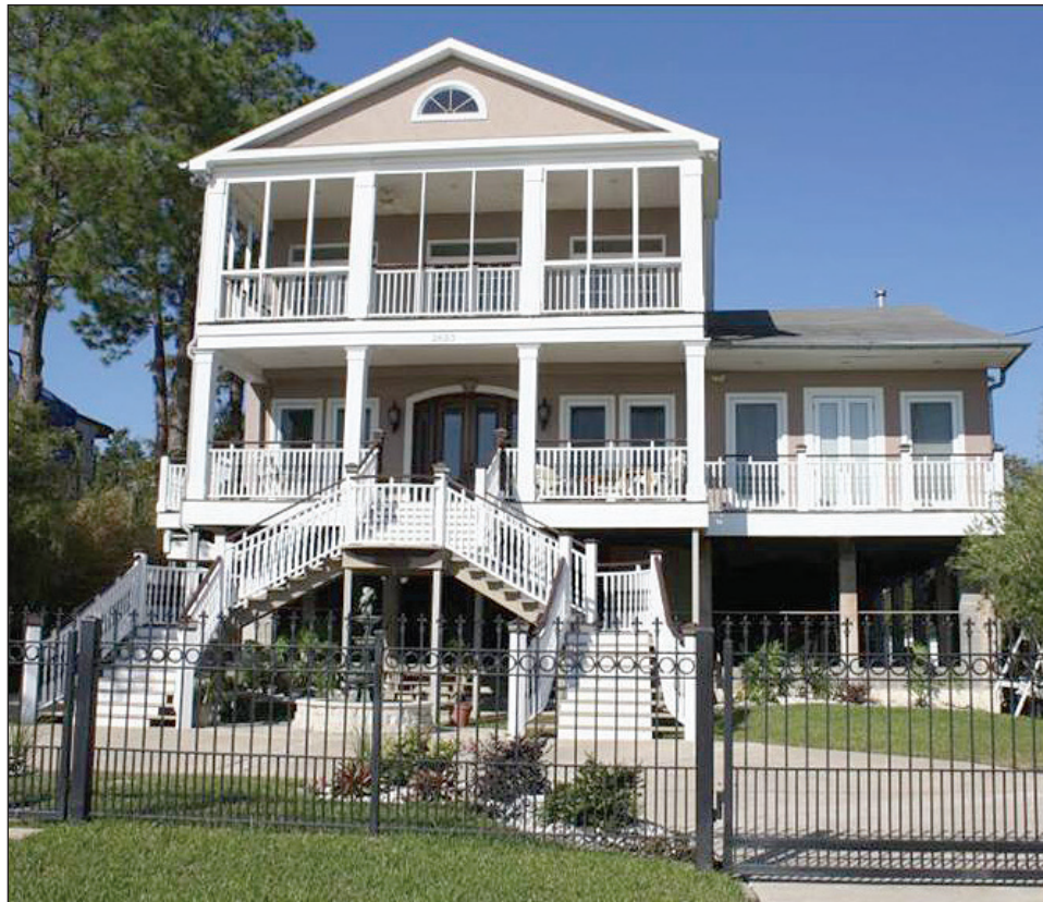
Figure 2-2. This home, from Figure 2-1, was elevated in a manner that added to both its appearance and its value. As a result of its elevation, the home avoided major damage from Hurricane Isaac in 2012.
