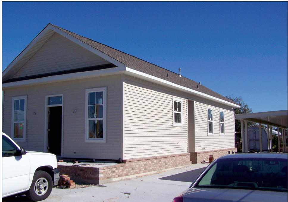
Figure 6-9. Typical mitigation reconstruction project.
